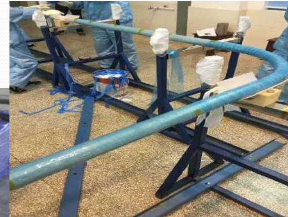
Silicon wrap to compress during curing
